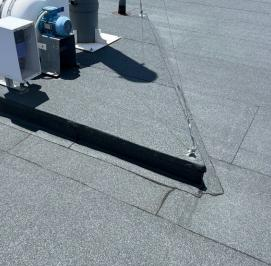
A triple-layer torch-on sheet membrane system provided a highly durable, UV-stable, long lasting waterproofing solution for the University of Queensland's Health Sciences building in Herston.
